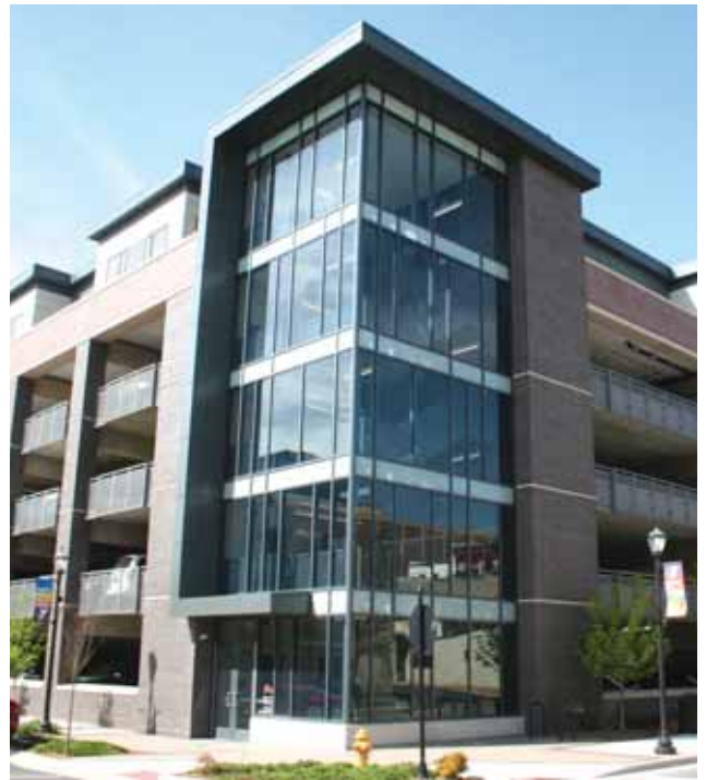
The cast-in-place concrete, post-tension parking garage in downtown Kokomo has one level on grade and four elevated stories.
