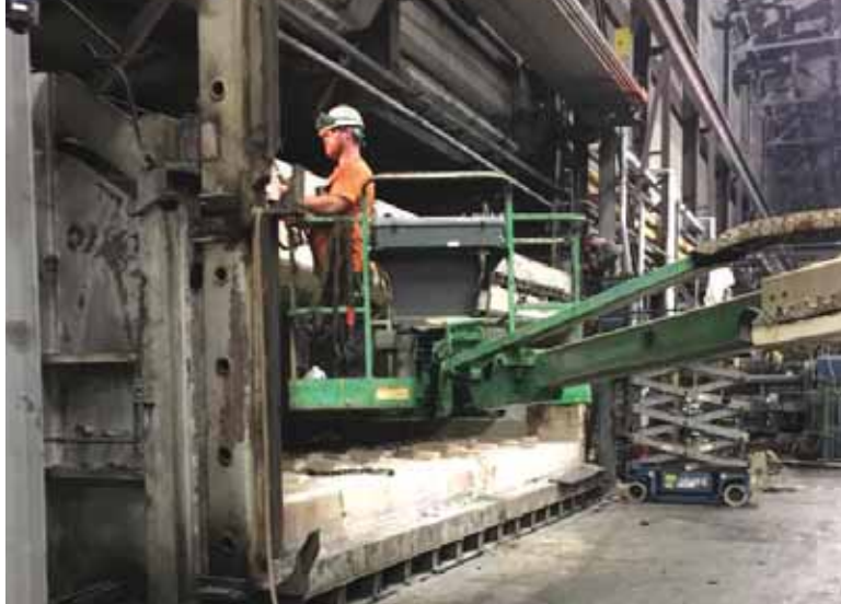
Apprentice Dain Hillis installs furnace doors at a steel mill in northeast Indiana.
